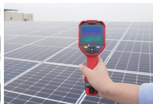
Solar panel Inspection
